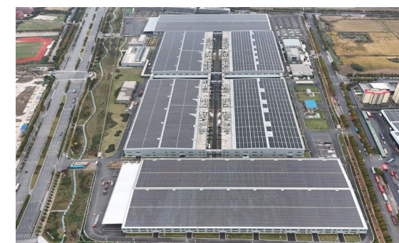
Wuhu LONGi Factory BIPV
