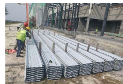
Processing Site of Roof Panels
