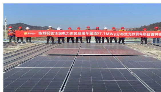
Grid Connection of Shiyang Dongfeng Commercial Vehicle Factory Project
