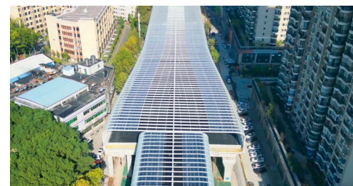
Sound Barrier Works of Wuhan Youyi Avenue Rapid Reconstruction Project
