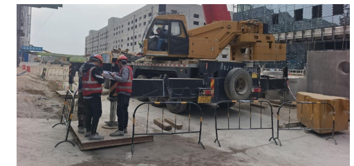
On-site Safety Inspection (Record)
