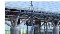
Modular Installation of Terminal Eaves
