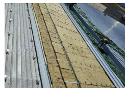
Installation Site of Roof Rock Wool
