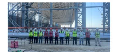
Noticeboard-announcing Acceptance of Hoisting Operation
