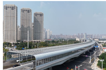
Sound Barrier Works of Wuhan Baishazhou Avenue Rapid Reconstruction Project
