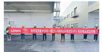
Grid Connection of Quzhou Jidian Three-Electric Intelligent Manufacturing Factory Phase I Project
