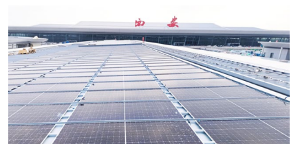
BIPV at Xi'an Xianyang International Airport
