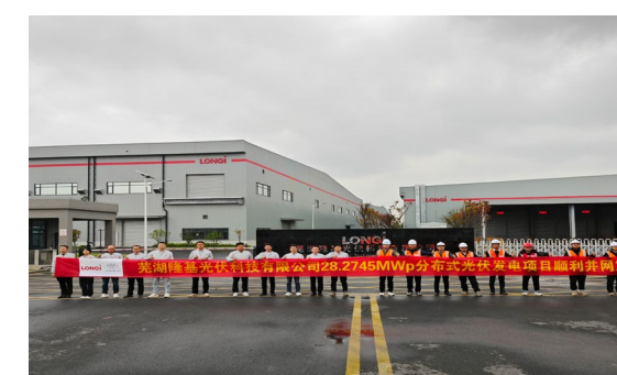
Grid Connection of Wuhu LONGi Factory Project
